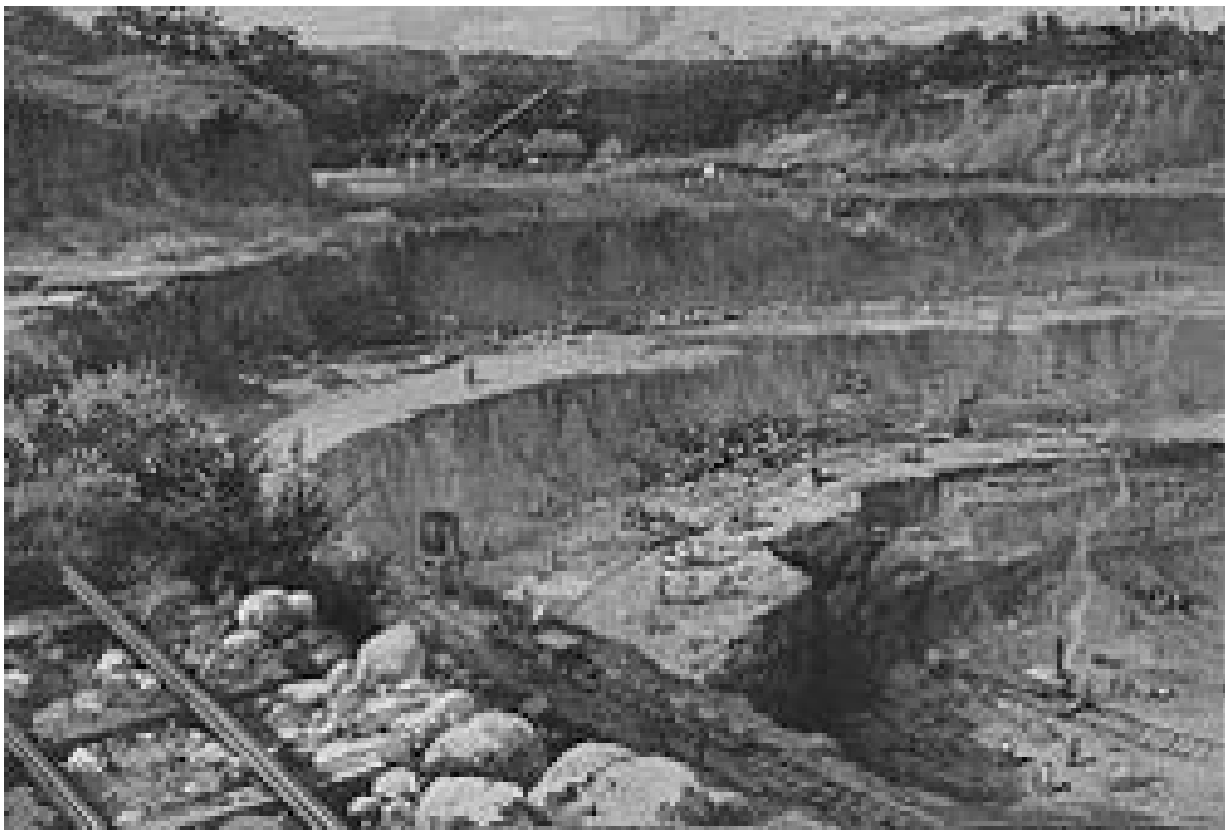
Figure 6 Excavation Work at Culebra Hill; note side slopes
