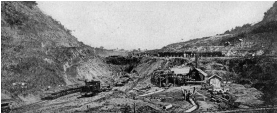
Figure 1 French canal excavation work at Cucaracha, 1885
